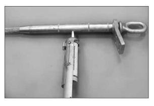
**Step #18** Cease application when filler compound seeps out the tapered "conductor facing" end of the hardware.
