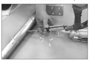
Step #22 While ensuring alignment of all hardware, insert the dead-end body into the compression press at the "Press First" knurl directly over the forged steel eye at the END of the aluminum body.
