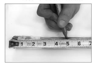
Step #4 Apply tape approximately 1" back from the cutting mark to secure the aluminum strands and maintain the conductor diameter after the cut is made.
