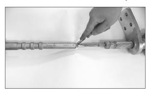
Step #9 Insert the steel core of the conductor into the bore of the steel dead-end eye. Make sure that the steel core goes to at least the mark or just past. Also ensure that roughly a 1" gap remains between the aluminum strands of the conductor and the edge of the steel dead-end eye as this allows room for material expansion underneath the press.
