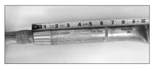
**Step #30** Mark the conductor with the measurement to ensure that the jumper is inserted to the adequate depth.
