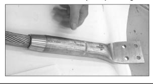
Step #35 Insert the jumper terminal into the press, and compress the conductor starting from the "Press First" knurl moving out to the edge of the tapered end of the tube.
