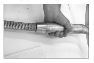
**Step #34** Ensure that the conductor is aligned and seated properly, and that the tab is facing the correct direction for your application.
