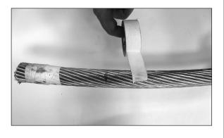
**Step #5** Cut the outer aluminum strands at the mark to expose the steel core.
