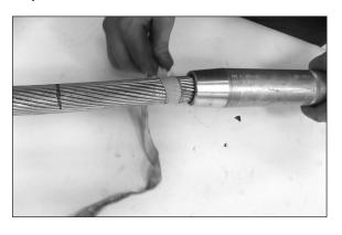
Step #32 Apply inhibitor (filler) compound to the aluminum conductor strands back to the mark. For ACSS Conductors, the inhibitor must be rated for temperatures up to 250°C.
