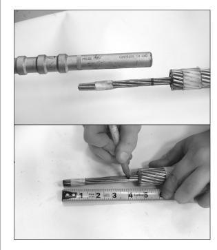
Step #7 Apply the aluminum dead-end body to the conductor starting with the tapered end and pushing the tube over the conductor slightly past the terminal tab.
