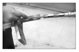
Step #16 Slide the aluminum body back against the felt washer and steel eye making sure to align the hardware properly.
