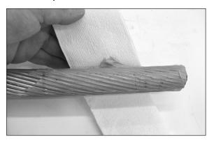
**Step #33** Insert the conductor fully into the jumper terminal.
