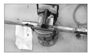
Step #25 Compress the conductor from the "Press First" knurl out towards the conductor, applying compressions all the way to the tapered end.
