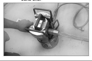
**Step #36** If desired by the utility, the jumper terminal may be rotated 90° for each succeeding compression until the end of the tube is reached.
