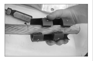
Step #27 If necessary, file down the conductor to ease insertion into the jumper terminal.
