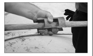
Step #2 Remove the plastic plug from the aluminum body. Inspect the inside bores of the hardware to ensure that there are no sharp points or other defects.
