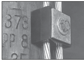
FIBERLIGN Downlead Cushion mounted to wood pole
