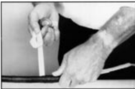
FIGURE 15 - APPLYING LOCK-TAPE SEALANT
