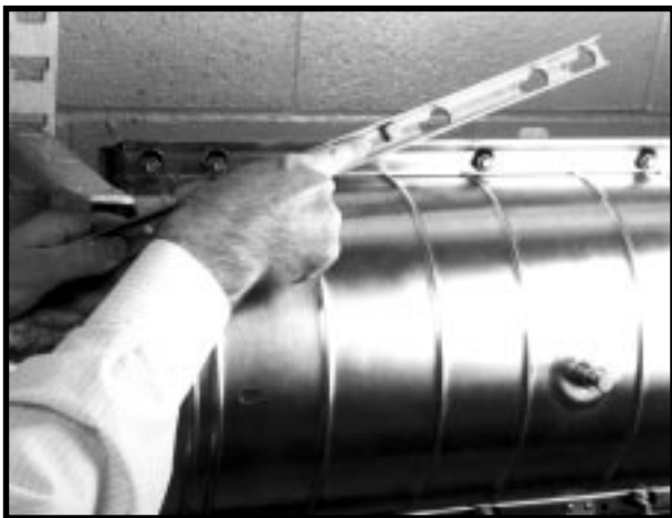
FIGURE 1 - PLACE SUPPLIED BOLT THROUGH HANGER HOLE
