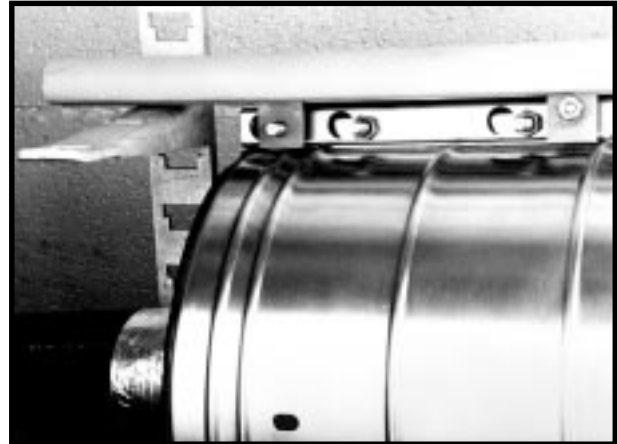
FIGURE 5 - PUSH SLIDER OVER REAR TEE
