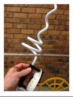
**Step #5** Holding the nylon swing tube and coil end directly under the line, wrap the PVC coil around the line snapping the tail into place.
