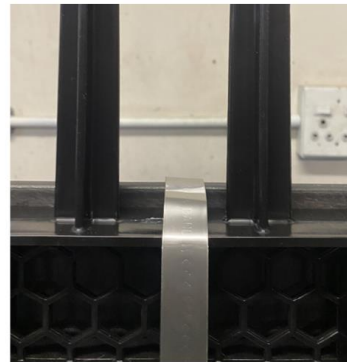
Stainless steel straps are fastened over the BG, through the verticals, and around the angle iron.
