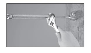
**Step #2** Extend the turnbuckle before taking the measurement for your strand length.
