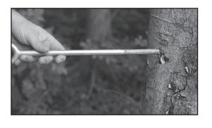
PLP Tip: Install the TREE-GRIP™ Dead-end, thimble, and cable. Tighten nut on the other side of the tree. Reference the TREE-GRIP Deadend application procedure (SP2056).
