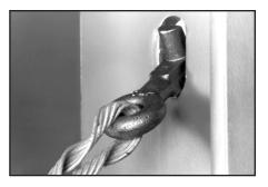
**Step 3** Pull the BRACE-EYE toward you until the "T" Section rests against the back of the web plate. The square neck locks the BRACE-EYE in place.
