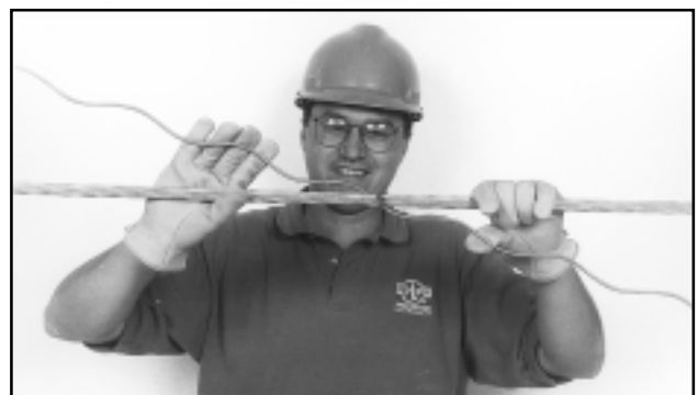
FIGURE 2 - APPLY AND WRAP FIRST ROD AROUND CABLE
