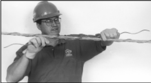
FIGURE 3 - APPLY REMAINING STRUCTURAL REINFORCING RODS
