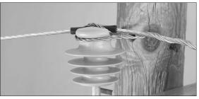
Step #6 Wrap the other leg of the Alloy Top Tie around the neck of the insulator.
