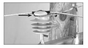
**Step #5** Continue wrapping to completion. Make sure to snap the end of the leg into place.
