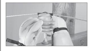
Step #4 Wrap the first leg (closest to you) tightly around the neck of the insulator.
