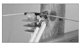
**Step #2** Align the Alloy Top Tie with the conductor as shown below, so that both legs are parallel to the conductor.
