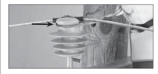
**Step #5** Continue to apply the first leg to completion. Make sure to snap the end of the leg into place.
