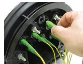
Installing Pigtail Connections
