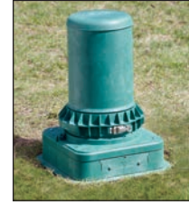
Installed 17" GLC with Grounding Spacer
