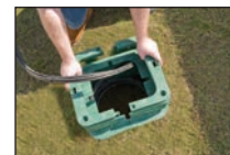
Spacer Installation
