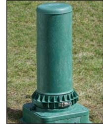
Installed 28" GLC with Grounding Spacer
