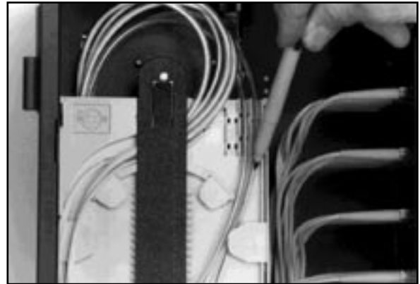
FIGURE 10 - MARK TUBES IN SPLICE TRAY
