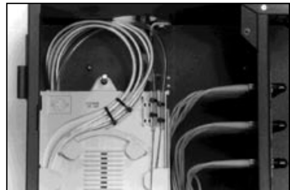
FIGURE 11 - SECURE TUBES TO SPLICE TRAY
