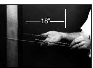
Step #1 Allow 18" from the inside of the stake to the center mark. Shown above is the VINE-LINE Connector ready to be installed.
