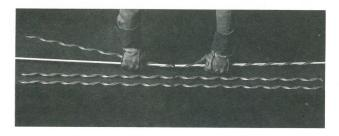
Hold the end of the second rod about ¼" away from the end of the first rod, as shown. Then completely apply the remaining length of the first subset.
