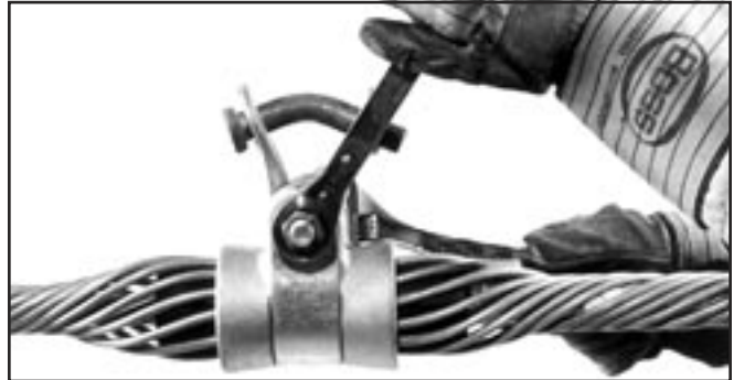
FIGURE 9 - APPLY LOCKING NUT AND TIGHTEN
