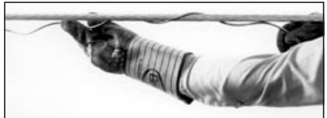
FIGURE 3 - APPLY ALL REMAINING INNER RODS AROUND THE CABLE
