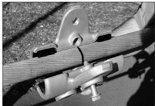
Install the clamp on the conductor.
