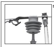
Step #4 It may be beneficial to have a pole buddy lift the conductor while the tube is pushed into place.
