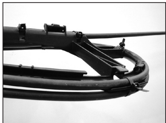
FIGURE 19B: CABLE SECURED TO EXPANSION TABS FOR 20" (508MM) LOOP - OVER & UNDER.
