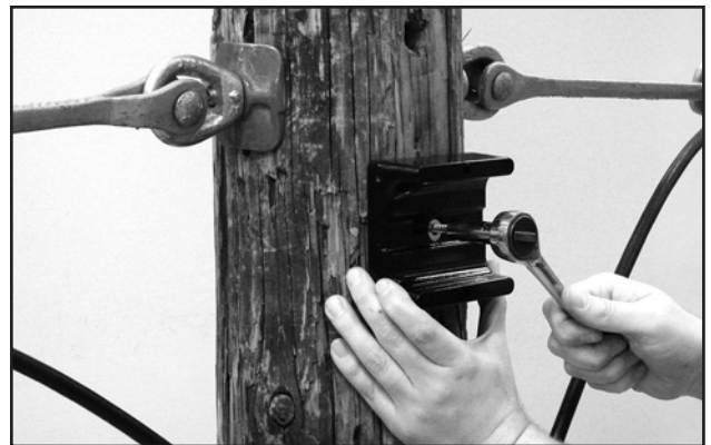
FIGURE 7: POSITION BACK HALF OF UCG AND SECURE WITH SHORT LAG SCREW
