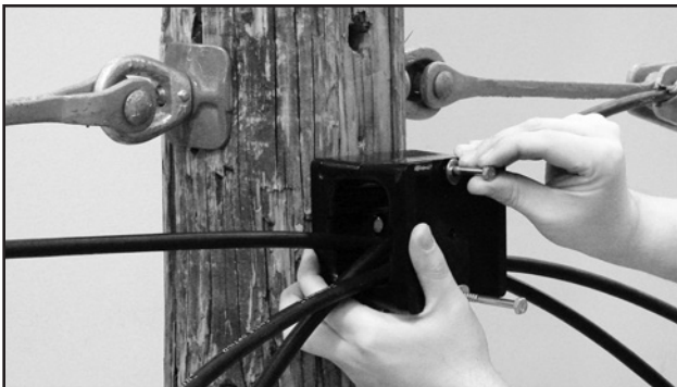
FIGURE 9: CAPTURE CABLES AND SECURE UCG FRONT HALF WITH TWO LONG LAG SCREWS
