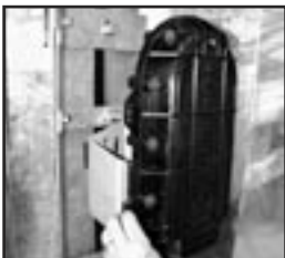
FIGURE 24 - INSTALL COYOTE RUNT ONTO VERTICAL MOUNTING BRACKET
