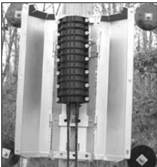
FIGURE 17 - DOORS INSTALLED
