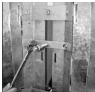
FIGURE 21 - INSTALL BRACKET CONNECTION ONTO FRAME
