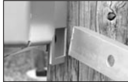
FIGURE 34 - RECTANGULAR FRAME HOLE ACCEPTS CROSS-ARM
