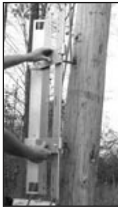
FIGURE 7 - HANG FRAME ON POLE
