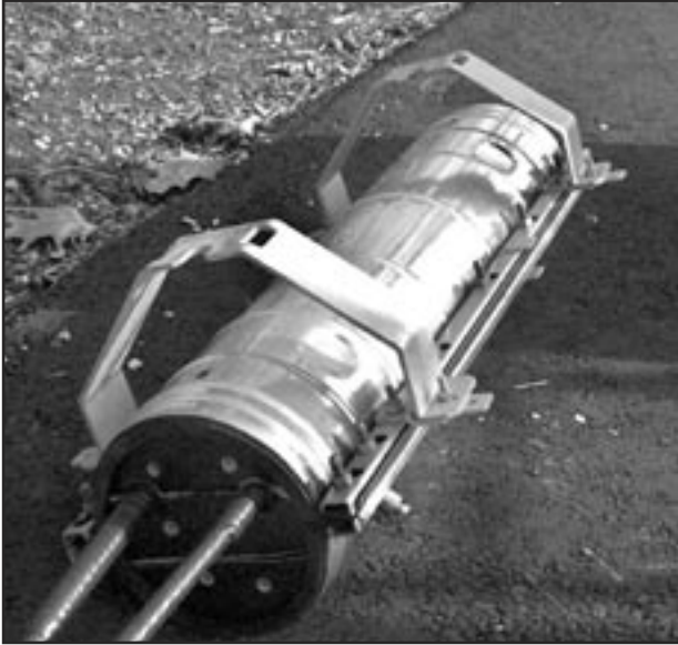
FIGURE 2 - SPLICE CASE VERTICAL MOUNTING BRACKETS
