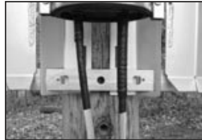
FIGURE 35 - SCREWS RETAIN CROSS-ARM
