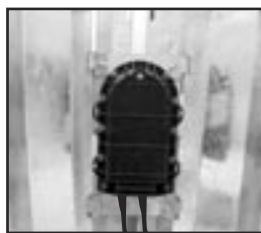
FIGURE 25 - COYOTE RUNT INSTALLED
