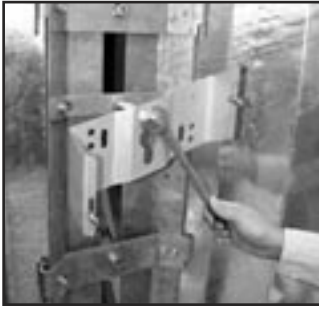
FIGURE 22: INSTALL VERTICAL MOUNTING BRACKET
