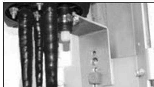
FIGURE 15 - HANG CLOSURE ONTO THROUGH BOLT.
