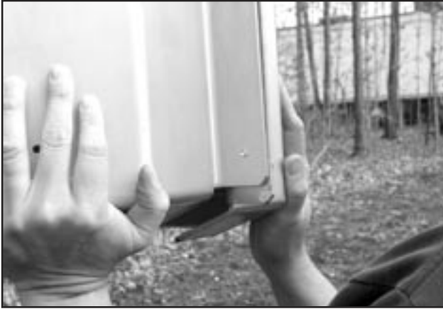
FIGURE 12 - LIFT ONE DOOR TO ENGAGE SCREW INTO OTHER DOOR
