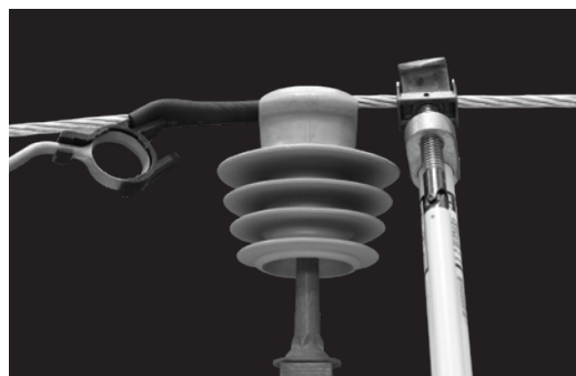
LIFT THE CONDUCTOR IF REQUIRED TO POSITION THE TUBE
