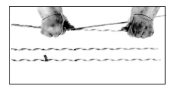
**3.00** Position second cut strand end against the first and completely apply remainder of subset. Do not exceed 1/4" (6 mm) separation of the strand ends.
