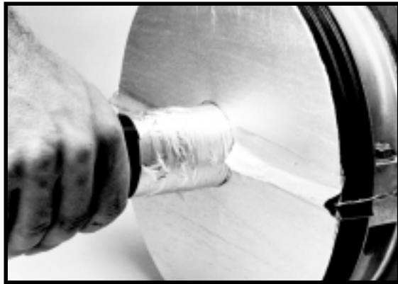
FIGURE 21 - HEAT SHIELD MATERIAL ON CABLE
