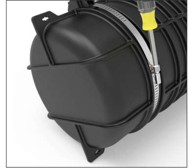
Installing Hose Clamp on COYOTE 9.5" Dome Closure
