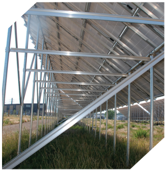
Underside of large ground mount
