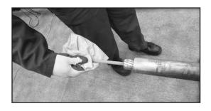
Step #5 Clean/wire-brush the entire aluminum area to be covered by the compression hardware per your standard company practices. Ensure that no residue or surface particles remain.
