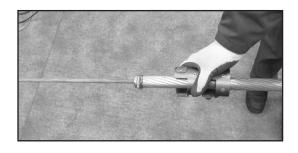
Step #6 Mark the conductor on Side A with the Filler Tube length plus 3/8" (10 mm) from the end of the aluminum strands.
