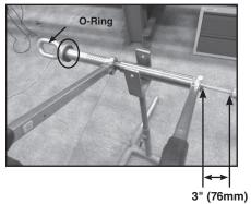
3" (76mm minimum Step #13 Slide the aluminum outer sleeve towards the eye, lining up the edge of the pad with the mark on the steel eye. If no mark is present, offset the deadend eye 1.6" (40 mm), as shown.
