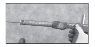
Step #7 With the tapered end of the inner aluminum sleeve facing the end of the conductor, slide it approximately 3 ft (1 meter) down the conductor.
