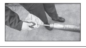
Step #5 Clean/wire-brush the entire aluminum area to be covered by the compression hardware per your standard company practices. Check that no residue or surface particles remain.
