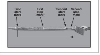
**Step #17** Compress the area marked on the outer aluminum tube closer to the eye, starting at the mark further from the eye. Compress until the o-ring is flush with the pad. Do not over compress and damage the o-ring. This should require 1-1/2 to 3 compressions to fully secure the dead-end.
