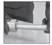
hardware (at least the length of the jumper inner aluminum sleeve) per your standard company practices. Check that no residue or surface particles remain. **Step #2** Apply the supplied oxide inhibitor along the length of the wire brushed aluminum strands.
