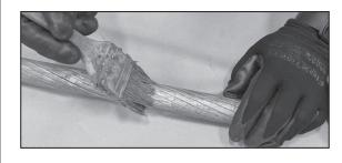
**Step #3** Use the supplied 220 grit sandpaper to lightly sand the outside of the inner aluminum sleeve.
