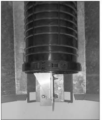
Completed Installation NOTE: When using the 9.5" x 28" Dome the bottom slots on the Defender for mounting the cable storage crossarm are not accessible and this crossarm should be mounted directly to the structure underneath the Defender.
