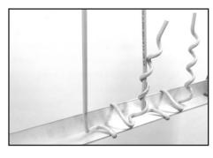
Step #6 Wrap the helical upright of the second deterrent around the straight upright of the first deterrent. Ensure that the bottom helical wrap is installed properly.
