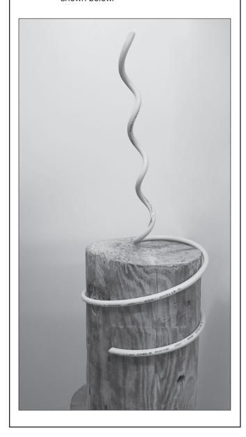
Step #2 Using ½ inch staples, secure the BIRD PERCH DETERRENT to the pole as shown below.
