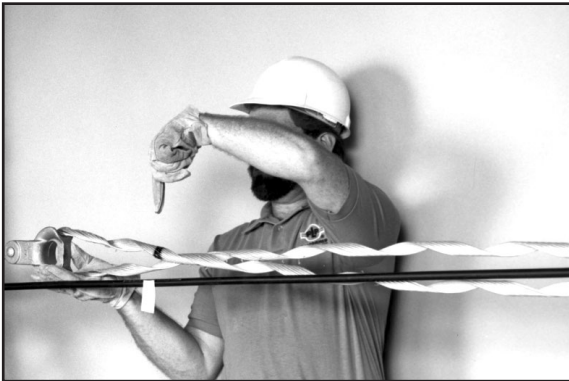
Positioning the THERMOLIGN DEAD-END
