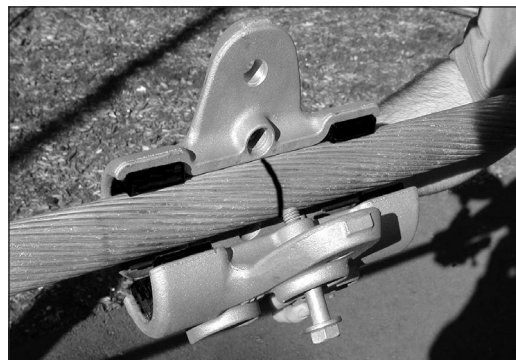
Install the clamp on the conductor.
