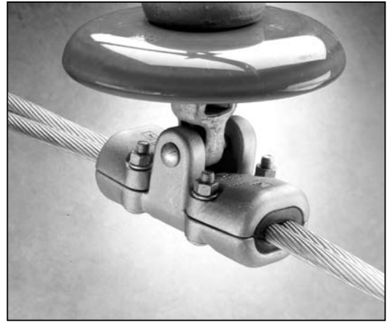
FIGURE 6 - COMPLETED INSTALLATION OF SUSPENSION CLAMP
