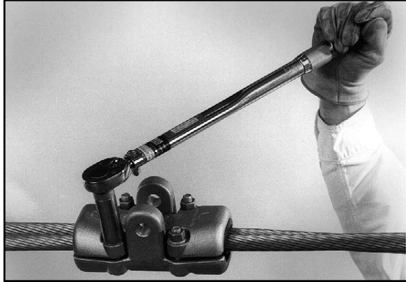
FIGURE 5 - TIGHTEN NUTS
