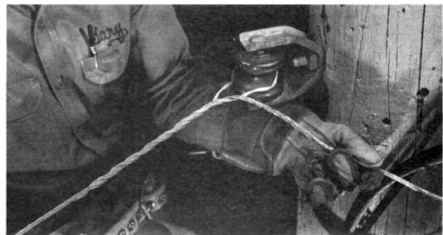
5. Completed application of the PREFORMED Service-Grip dead-end.
