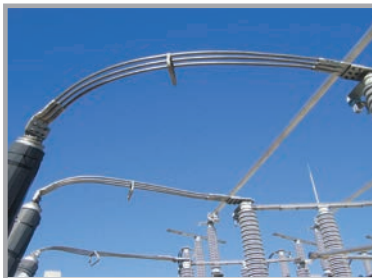
Aluminum Flexible Connector
