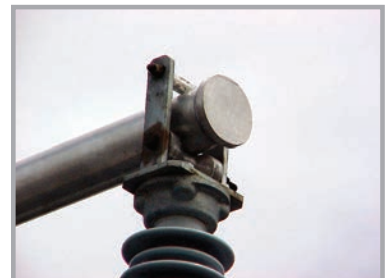
Busbar End Caps
