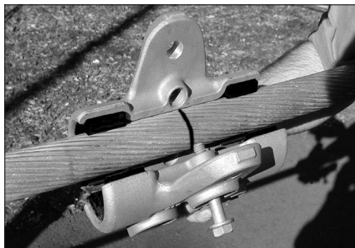
Install the clamp on the conductor.
