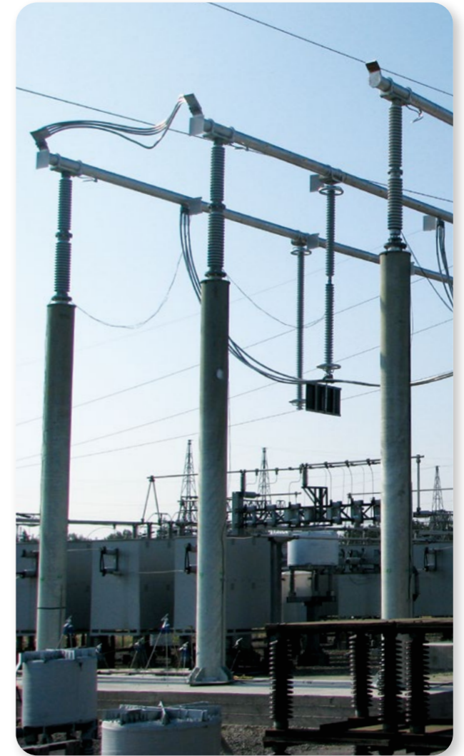
Full scale short circuit testing to 63kA/1sec.
