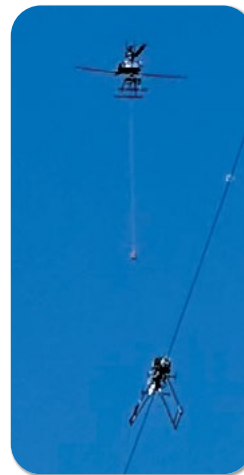
FulcrumAir E2500HP drone with FulcrumAir-PLP LineFly robot installing PLP Robot Bird Flight Diverters onto PEC transmission power lines.
