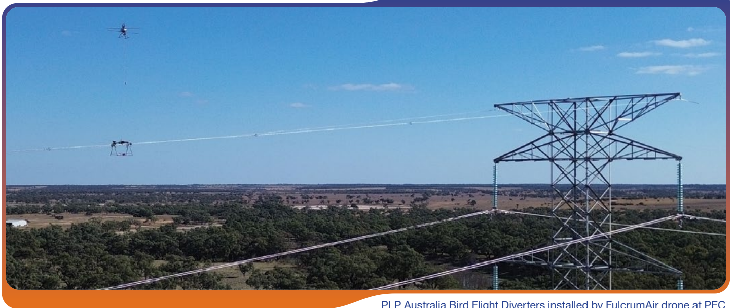
PLP Australia Bird Flight Diverters installed by FulcrumAir drone at PEC
