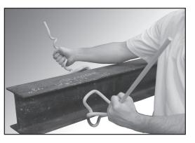
**Step #2** Keeping the uprights of the BIRD PERCH DETERRENT apart, position the unit so that the hooks are over the top of the I-Beam.
