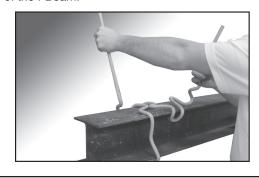
**Step #4** Install a second BIRD PERCH DETERRENT in the same manner as in Steps 1-3. Install the second BIRD PERCH DETERRENT with the uprights oriented the same way as the first BIRD PERCH DETERRENT.
