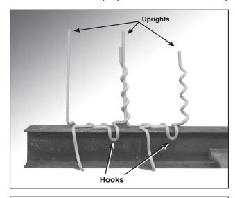
**Step #1** Spread the vertical uprights of the BIRD PERCH DETERRENT to position them around the I-Beam.
