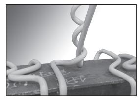
Step #6 Continue wrapping the helical leg until it is completely installed.
