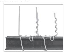
**Step #5** Wrap the helical upright of the first deterrent around the straight upright of the second deterrent. Ensure that the bottom helical wrap is installed properly.
