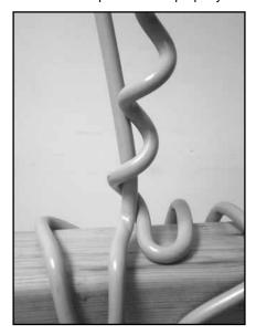
Step #7 Continue wrapping the helical leg until it is completely installed.
