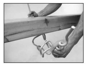
Step #2 Keeping the uprights of the BIRD PERCH DETERRENT apart, position the unit so that the hooks are over the top of the crossarm.
