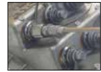
OptiTap Cable plugged into Terminal Closure
