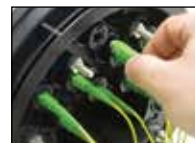
Installing Pigtail Connections
