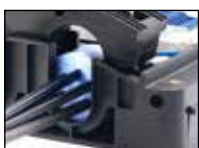
End Plate Installation
