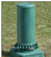
Installed 28" (749 mm) GLC with Grounding Spacer
