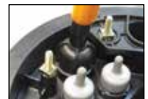
Field Installation of Hardened Adapter
