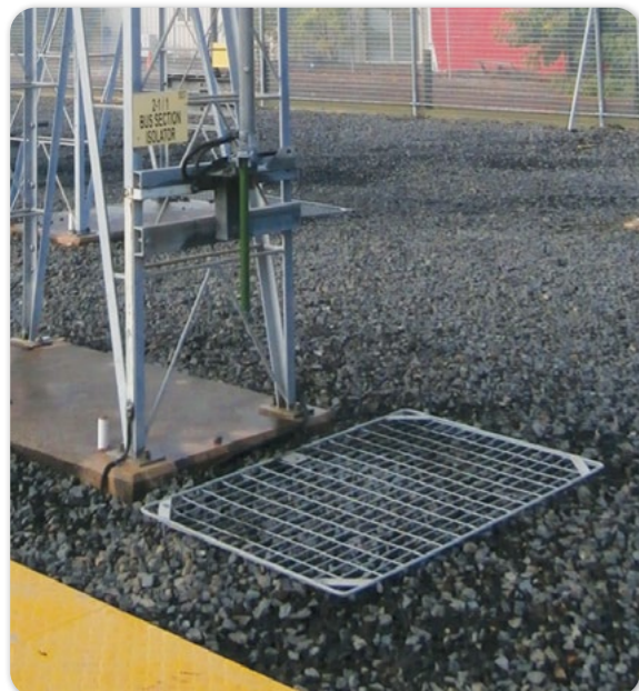
Installation of galvanised steel earth mat and kit
