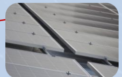
PV Module with Kliplok Clamp
