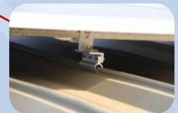
Metal Sheet Roof with Kliplok clamps
